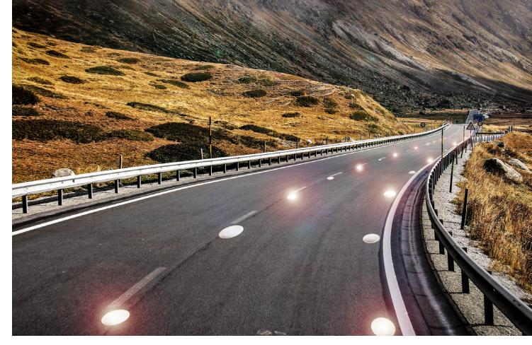
An example of a nudge that help drivers to slow down speed by providing an illusion of lights moving towards the driver.
