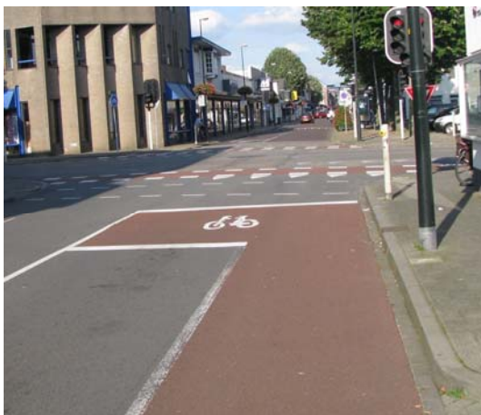
Figure 8: Example of a bike box (left) and a pre-start for cyclists, i.e. through cyclists have a green light while the light for right turning motor vehicles is still red (right)
