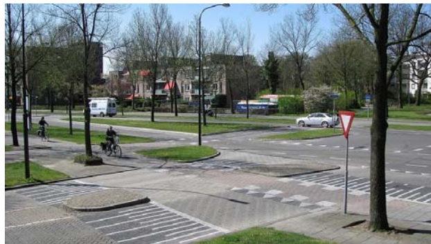
Figure 7: Example of an intersection treatment: a speed hump and clearance of 5m between the bicycle path and distributor road [43]
